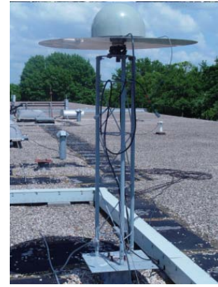
Fig. 6 Configuration of the ground plane test case at the AUT site.
